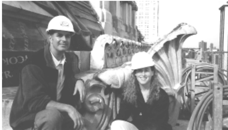
Jim Jamieson, Capitol Architect, showed HAF Executive Director Elizabeth Griffin around the roof re-construction site this fall.
