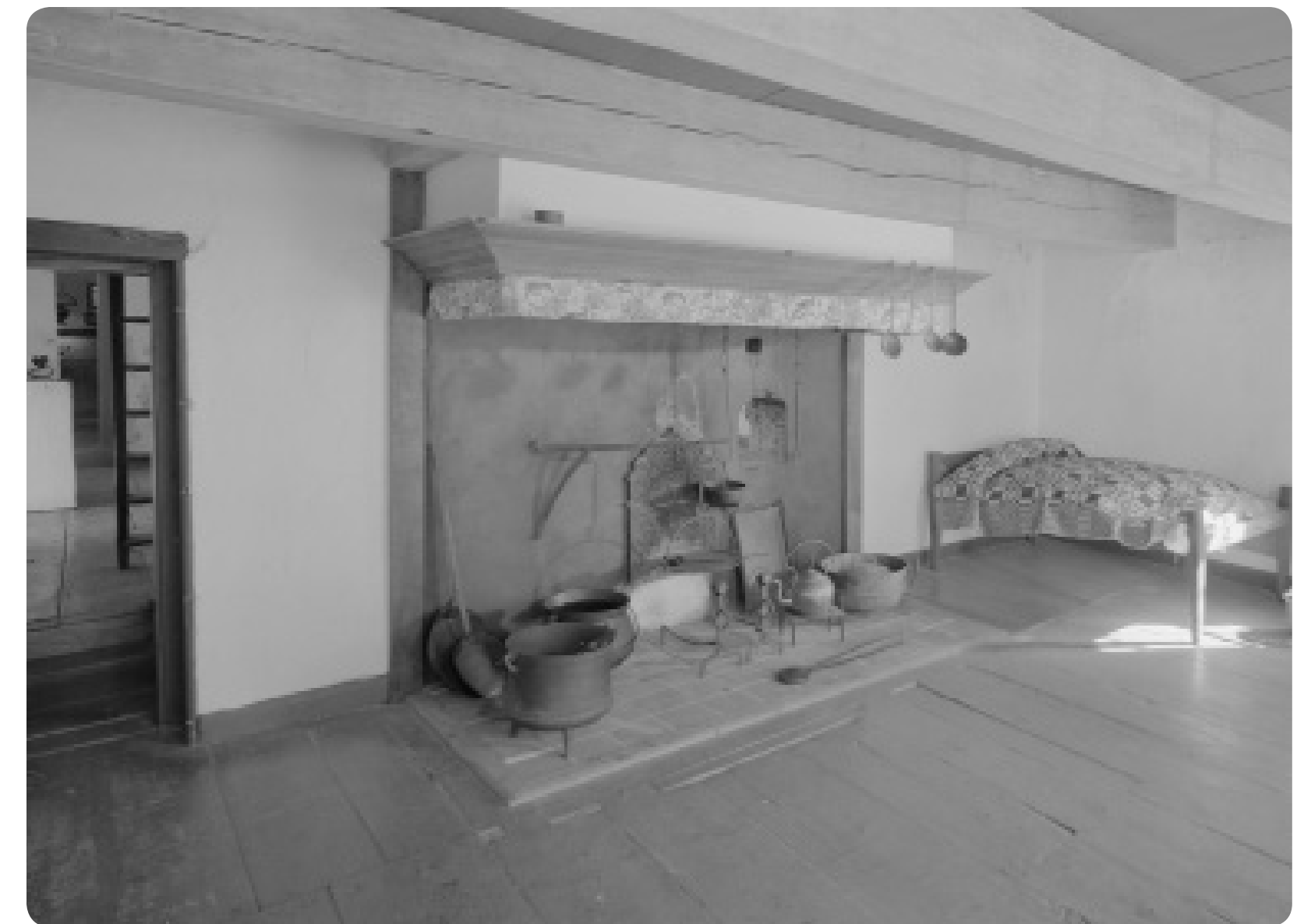
The replacement jambless fireplace from the Bevier-Elting House, Huguenot Street & Broadhead Avenue, in New Paltz. Library of Congress, Prints & Photographs Division, HABS, HABS NY,56-NEWP, 2--9
